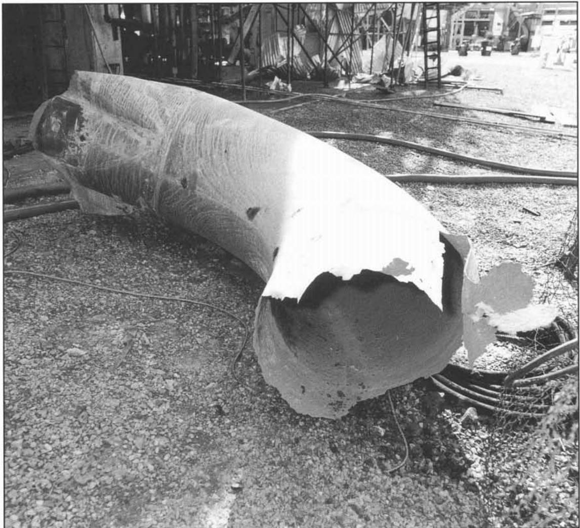
Figure 5 The 30 inch flare line elbow bend that failed and fell to the ground, releasing the hydrocarbon liquid and vapour
