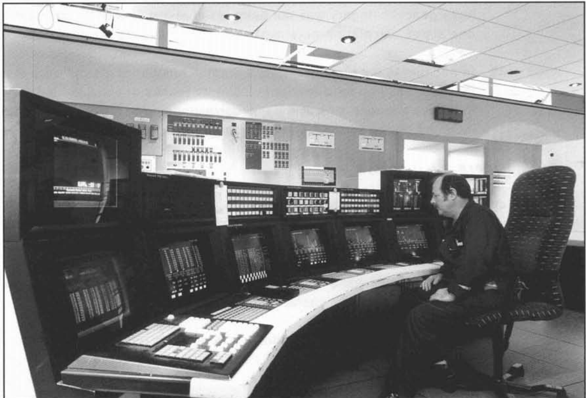
Figure 3 Part of the main control room, showing the display screens and keyboards used to operate the plant
